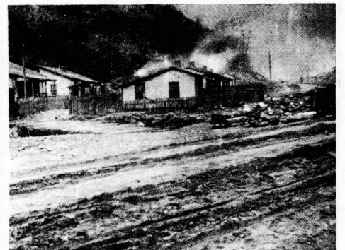
Scene at Wallins Creek, Ky. Miners' shacks.
