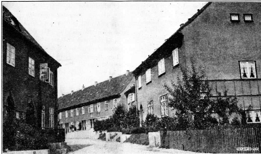
WORK OF THE PAINTING GUILD House Erected by the Building Co-operatives of Hamburg
