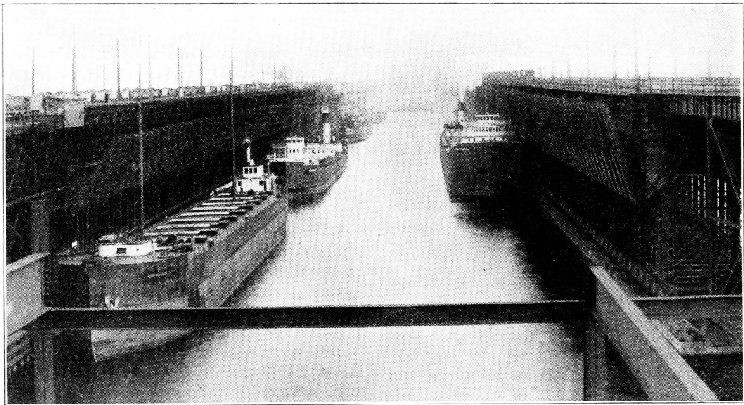
THE GREAT ORE DOCKS AT DULUTH. MANY A MAN HAS MET DEATH BY SLIPPING OFF THE NARROW DUMPING PLATFORM IN ICY WEATHER. THE ORE IS DUMPED FROM THE CARS ON TOP DIRECT INTO HOLDS OF THE ORE BOATS
