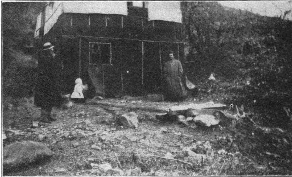
A TYPICAL "JUNGLE TOWN" HOME WITH THE WINDOW PANES MISSING.
