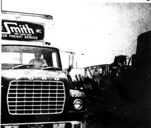
Wreckage of burned-out Earl C. Smith terminal in background.
