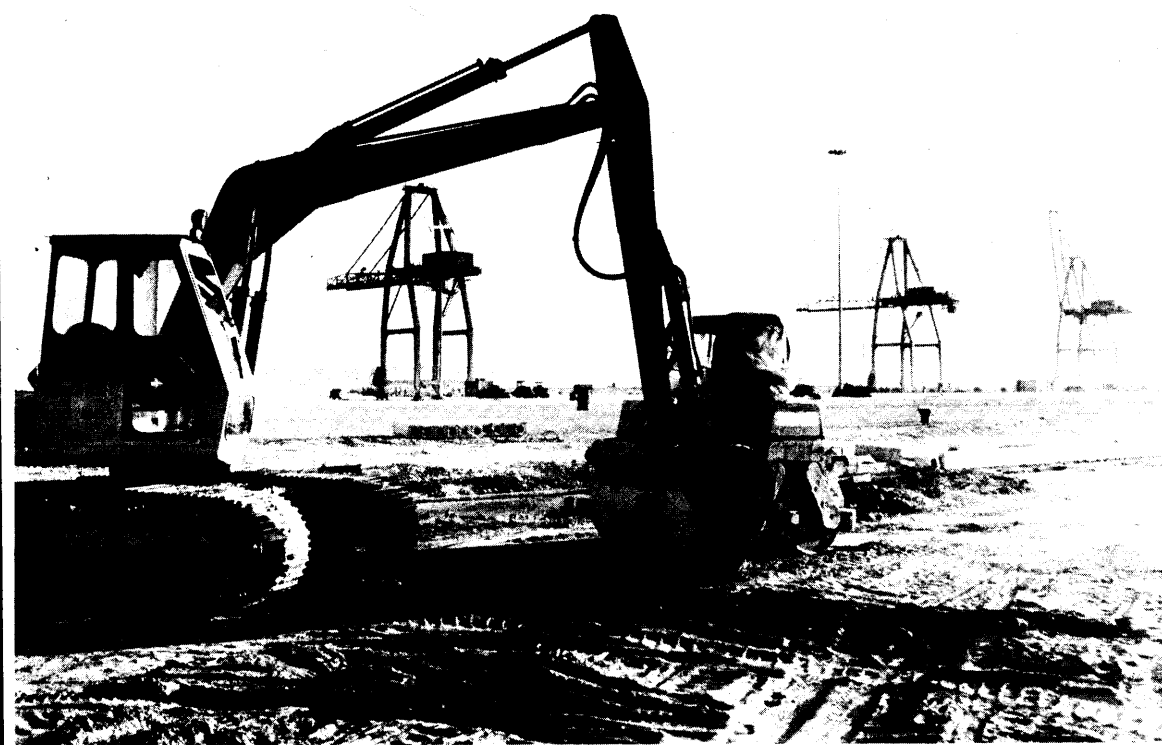
The nearly-completed Seaforth container terminal on Merseyside where dockers yesterday extended the black on handling containers.
