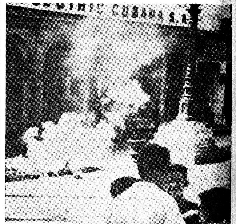
Flames shoot from a gas main, broken during street fighting in Havana in last month's abortive Castro-led revolution against Batista's dictatorship. Cuban government sources claimed at least 40 rebels were killed in the capital. Most of Havana population did not support the rising.
