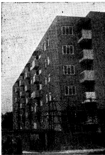
Working class flats under construction on the L.C.C.'s Lansbury Estate, Poplar.
