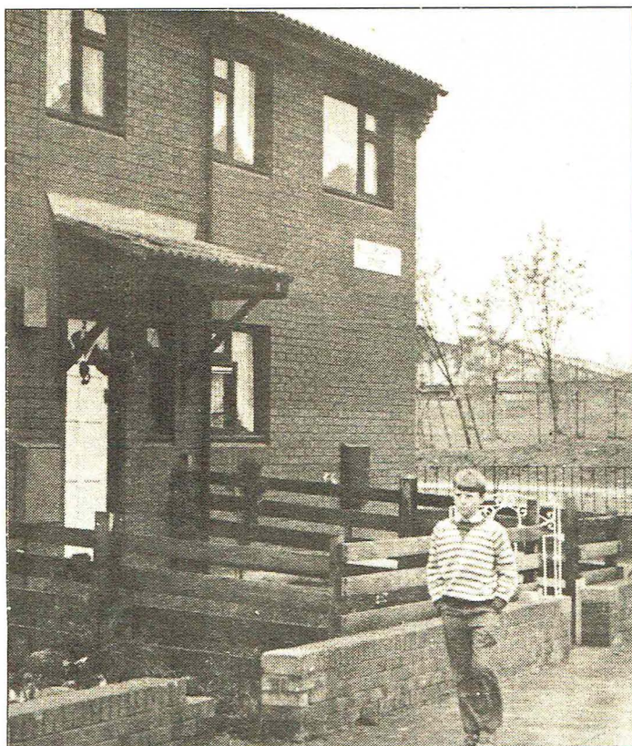
New houses with gardens built by Liverpool council according to Liverpool district Labour Party policy.
