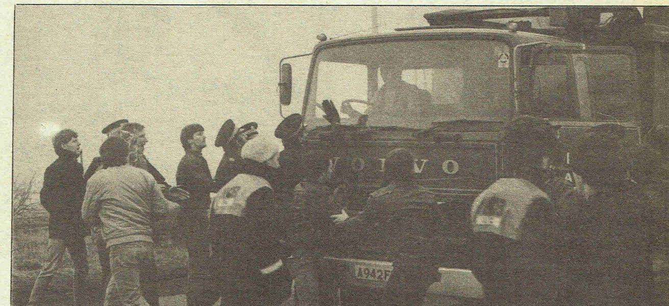
Pickets at Longannet Power Station in Fife.
