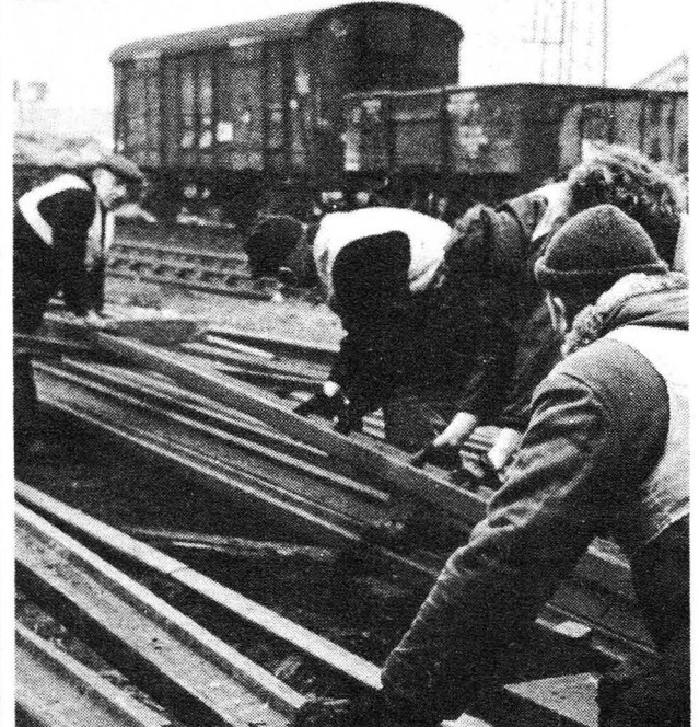
Cuts in maintenance—and therefore safety standards. The report says safety standards are 'too high'!
