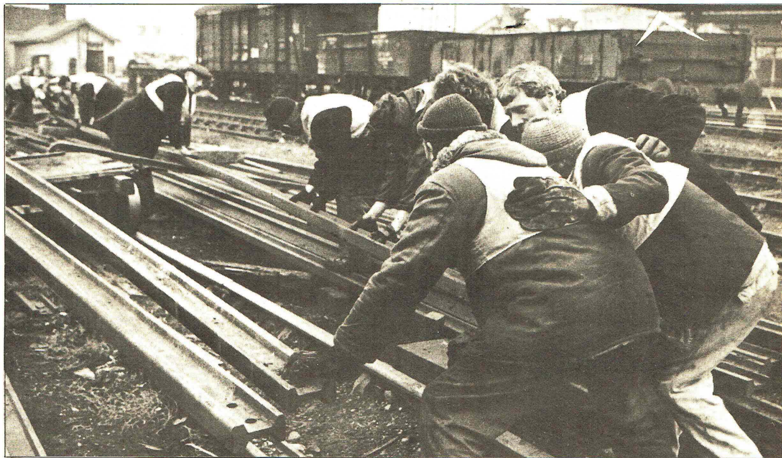
Laying track in Tyne yard
