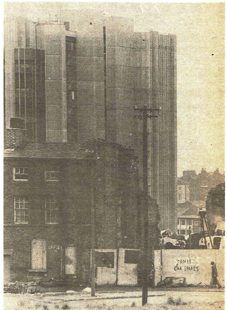
Houses are left to crumble away while the skyline is dominated by office blocks, many of which are left empty for years by property speculators.
