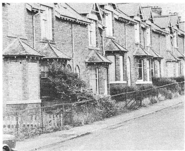
A typical scene in Newtongrange—house after house bricked up by the NCB
