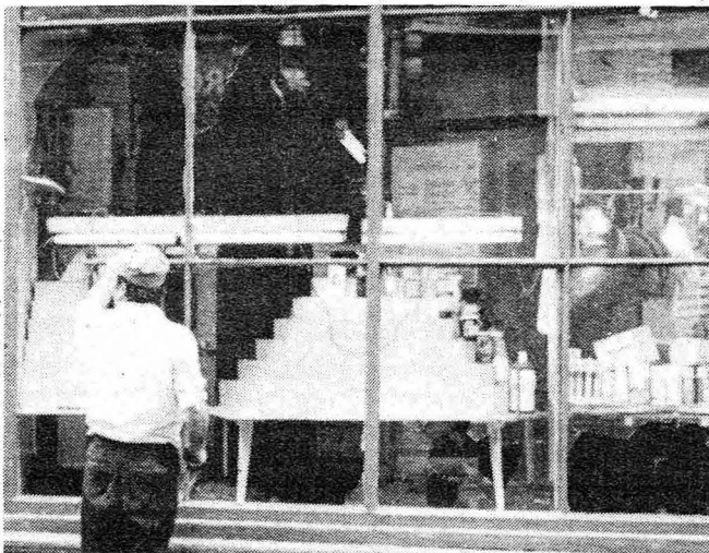
Repairing smashed windows after fascist rampage in Brick Lane
